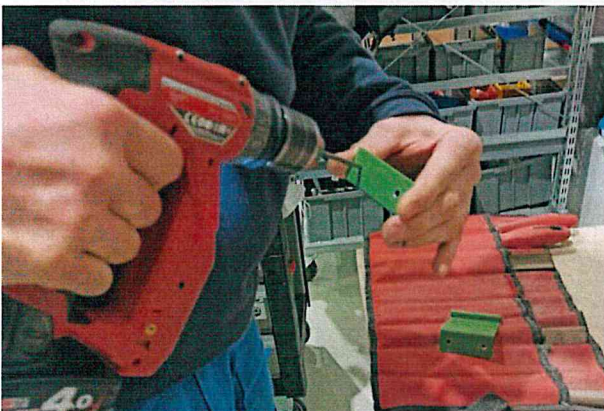
Redrill holes through the new brackets using 5mm drill bit.
